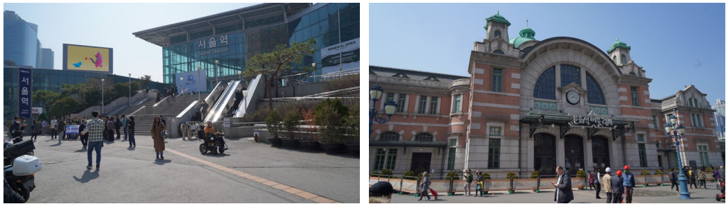
The new Seoul Station (left) and the old station “Culture Station Seoul 284” (right)
